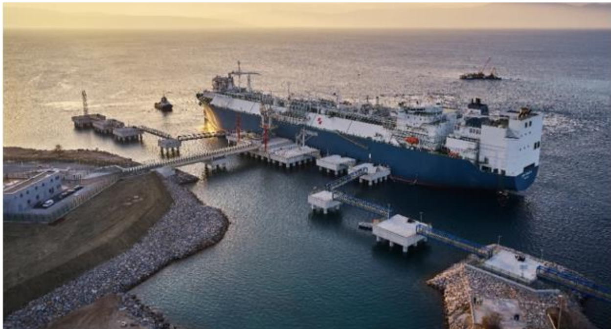
Figure 2. LNG terminal on the Island of Krk 9
